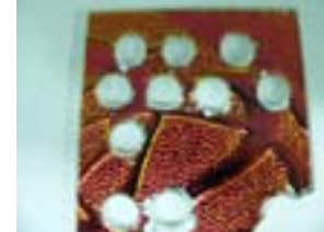
Many holes in one tile using this method. Note the cracked corner.
